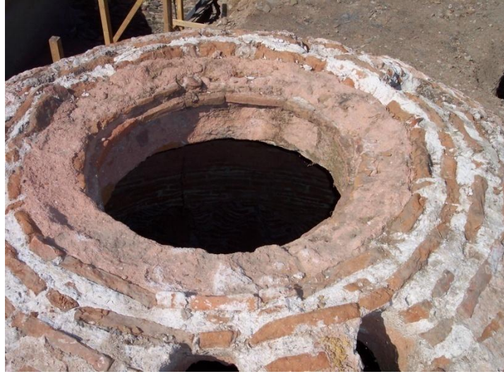
Figure 3.44. The use of lighting cupola in the northeast halvet domes of Tire Tahtakale Hamamı.
