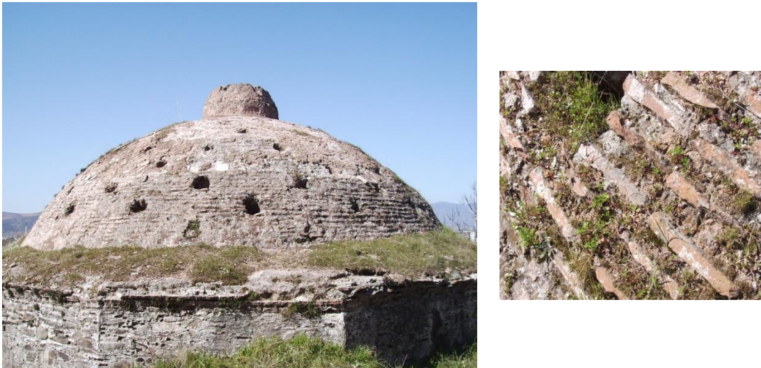
Figure 3.27. In Tire Yalınayak Hamamı men's section sıcaklık main space dome using the bond type of “horizontal stacking of long faces on the bottom for a few rows and short faces on top in parallel rows”.
