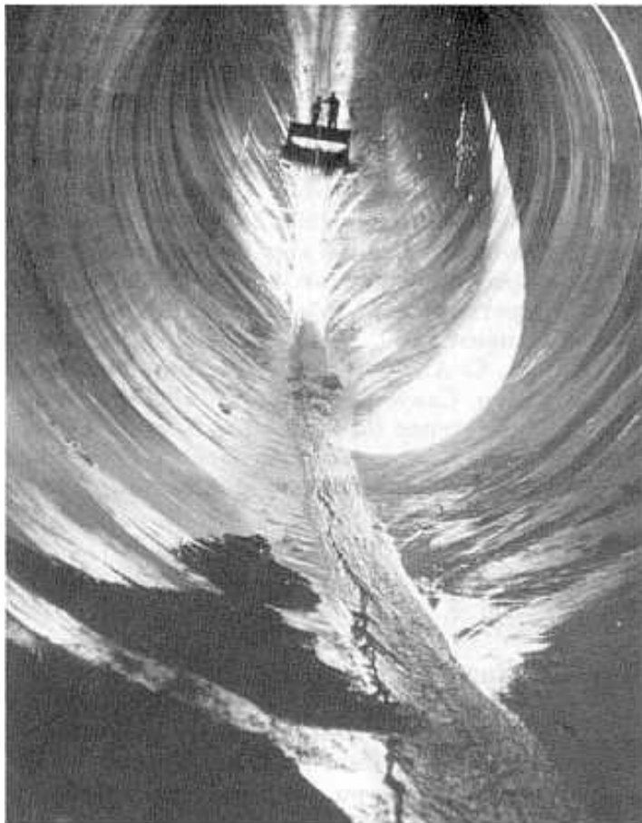
Figure 5.9: Yellowtail Dam, tunnel spillway - damage in elbow (Falvey, 1990)
