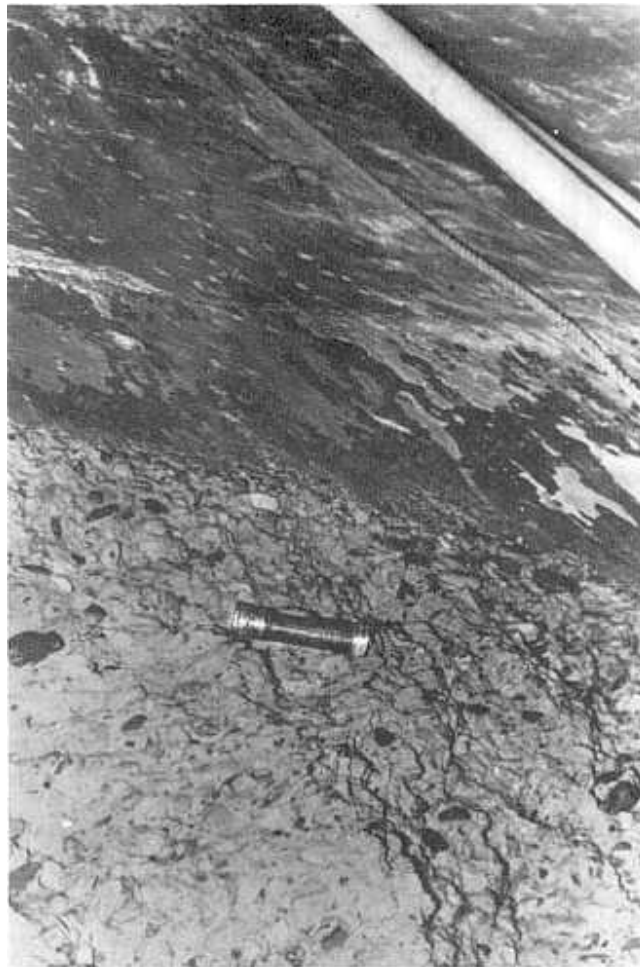
Figure 5.6: Hoover Dam, Arizona tunnel spillway-misalignment that caused major damage (Falvey, 1990).
