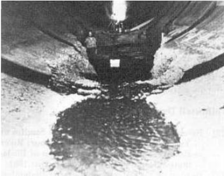
Figure 5.8: Yellowtail Dam, tunnel spillway-major damage downstream of elbow (Falvey, 1990)
