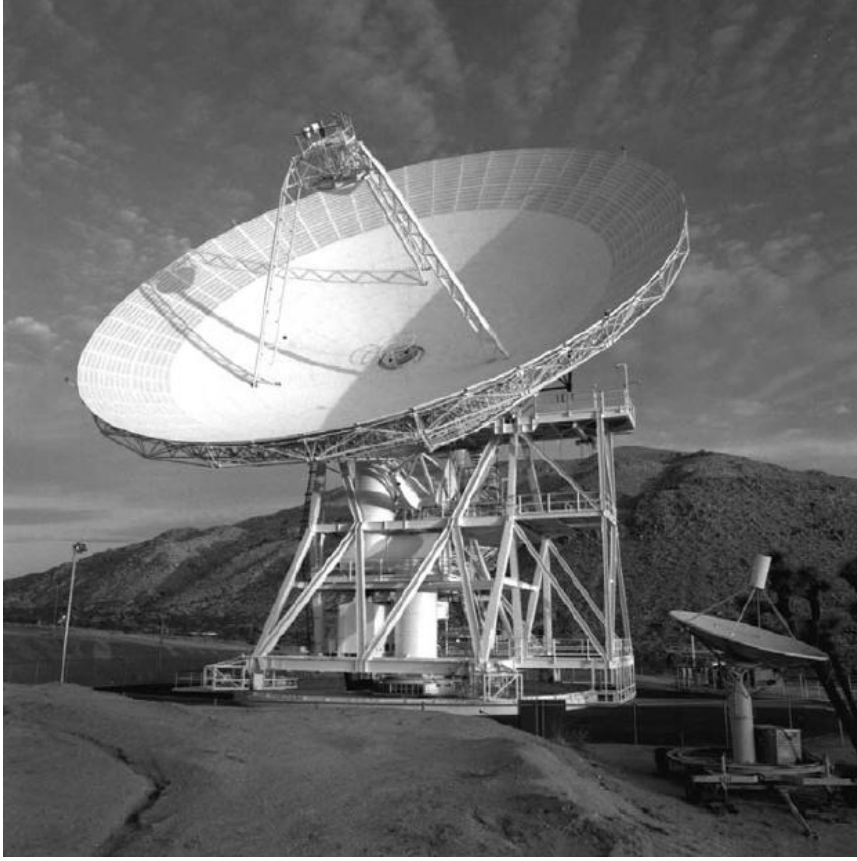
Şekil 1.7 Deep Space Network Anten, Goldstone, California
