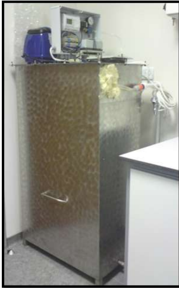
Figure 3.2. MicroClear® MBR for Greywater Treatment
