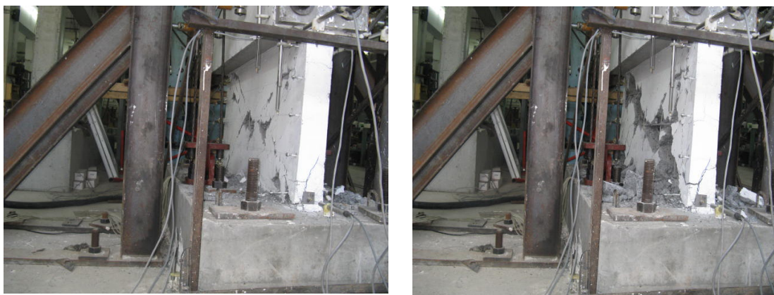
Figure 3.27. Medium and High Damage Levels (T1-N5-S1).
