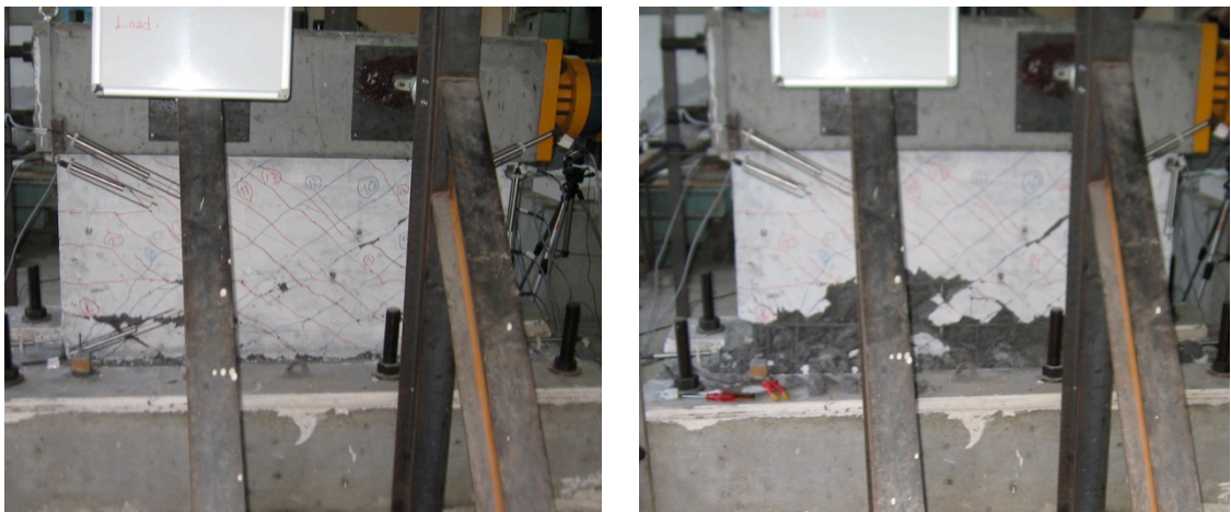
Figure 3.12. Medium and High Damage Levels (T2-S3).
