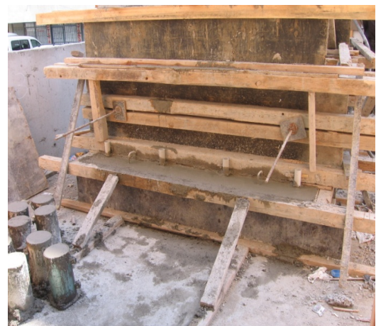
Figure 2.20. Freshly-cast concrete and cylinder specimens.
