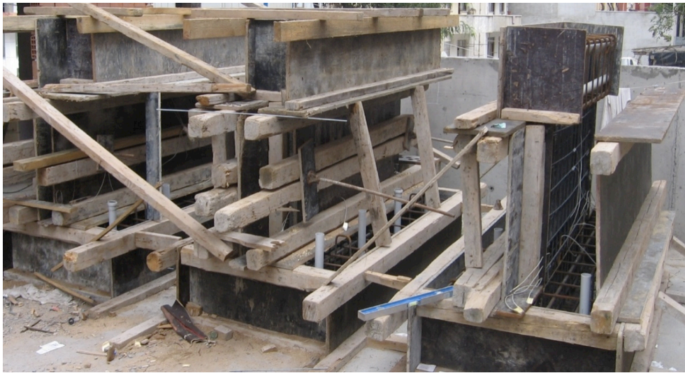
Figure 2.19. Shoring of the Formwork.
