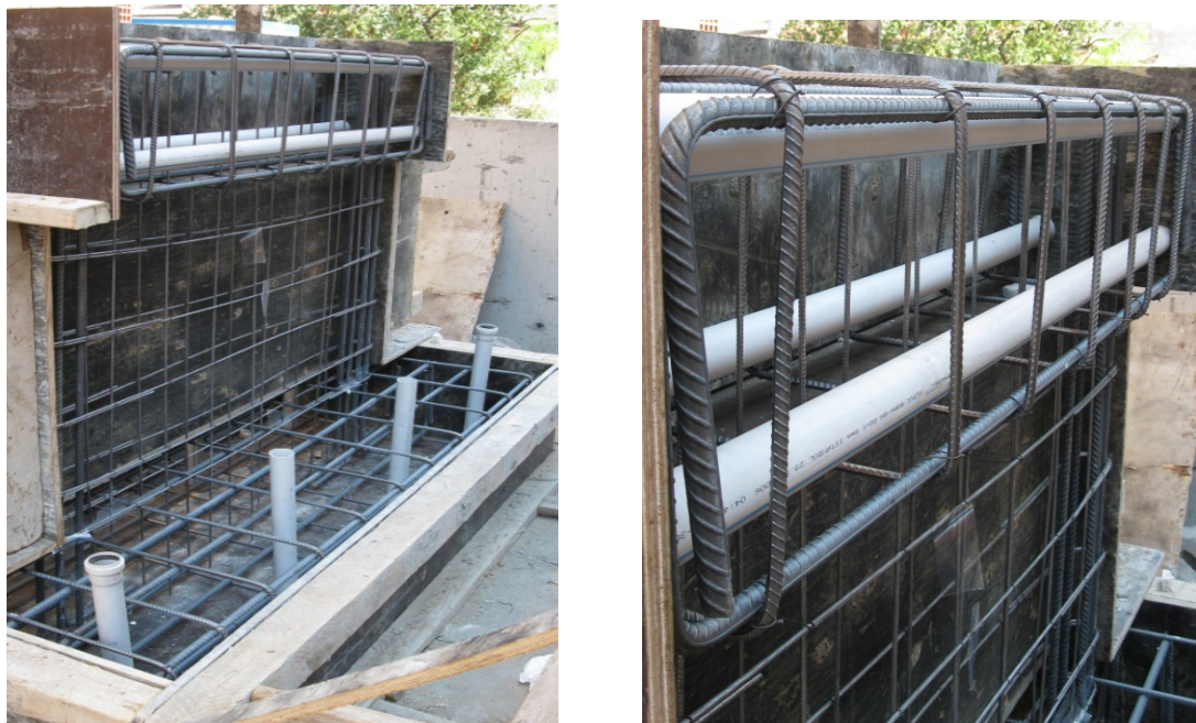
Figure 2.17. Formwork and reinforcement of Beam.
