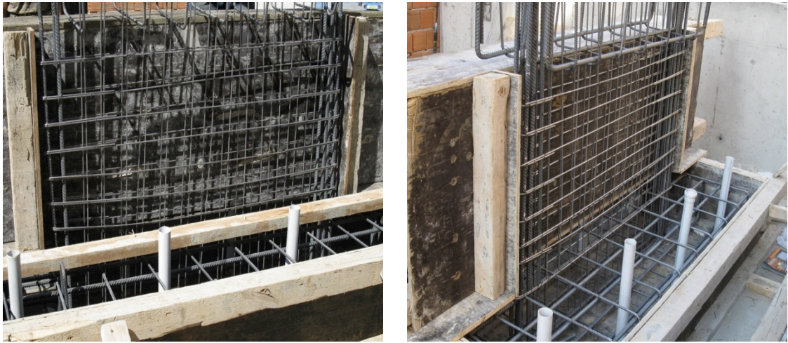
Figure 2.16. Wall and Beam Reinforcement.
