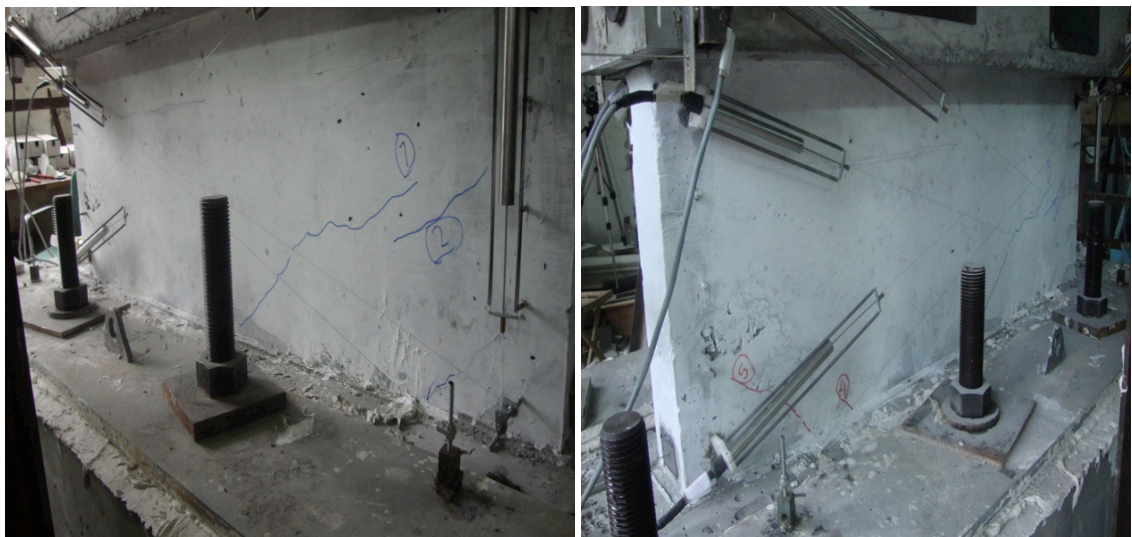
Figure 3.16. Initial Diagonal Cracks (T4-S1).
