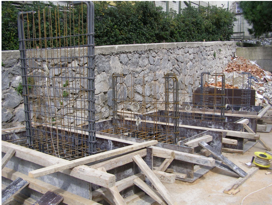
Figure 2.22. Bottom Pedestal Formwork and Wall Reinforcement.
