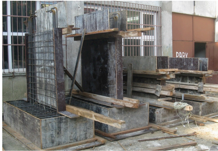
Figure 2.21. Construction of the second set of specimens.
