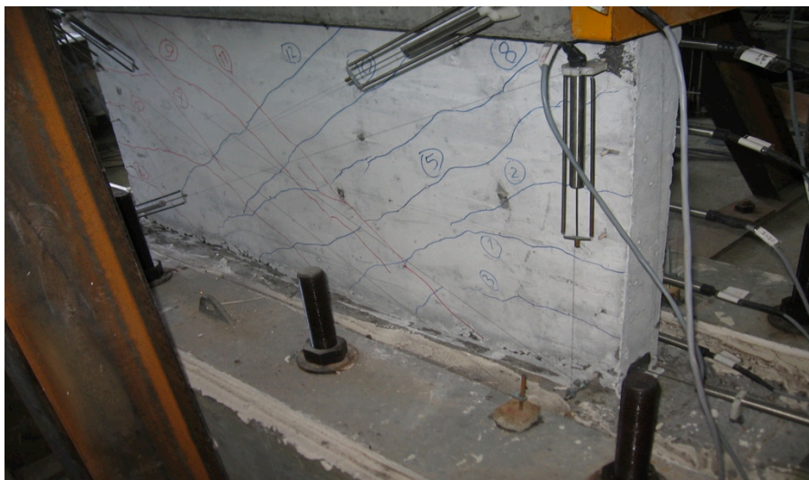
Figure 3.11. Cracking Pattern at Ultimate Load Level (T2-S3).
