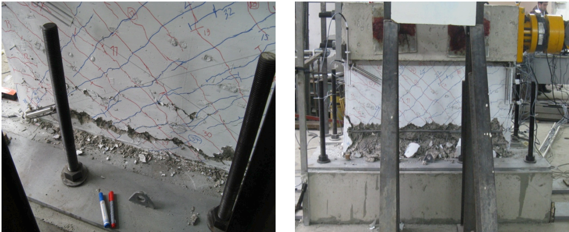
Figure 3.6. Medium and High Damage Levels (T2-S1).
