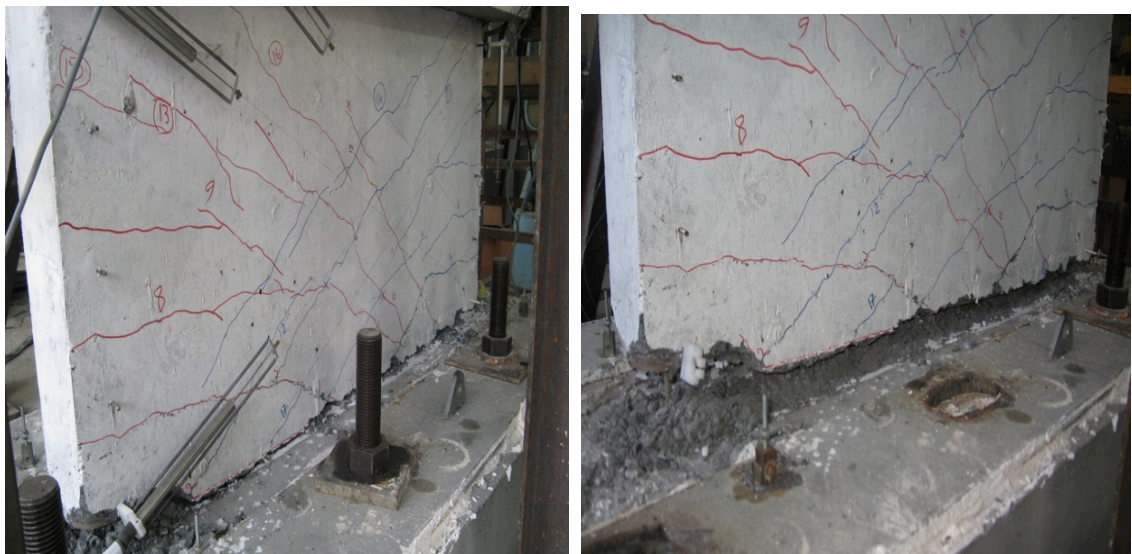
Figure 3.15. Medium and High Damage Level (T3-S1).
