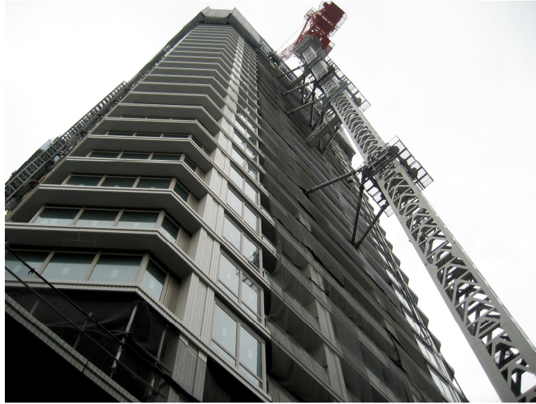
Figure 2.16 The Nabeaura Tower in Yokohoma, Japan uses precast ECC coupling beams in building core for seismic resistance
