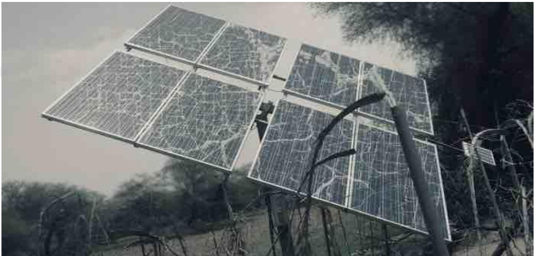
Figure 1.9. Solar panel system in early 1900's (makeuseof.com, 2015).
