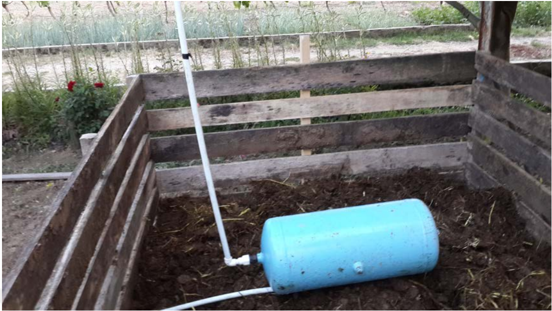
Figure 2.15 Water tank inside compost reactor II –Turkey (Personal archive, 2017)
