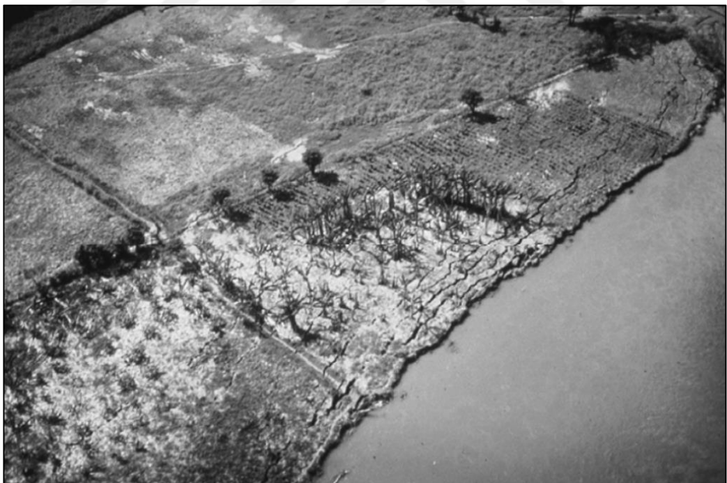
Figure 2.3 Lateral spreading of very flat ground toward the Motagua River following the 1976 Guatemala earthquake. Note orientation of ground surface cracks parallel
