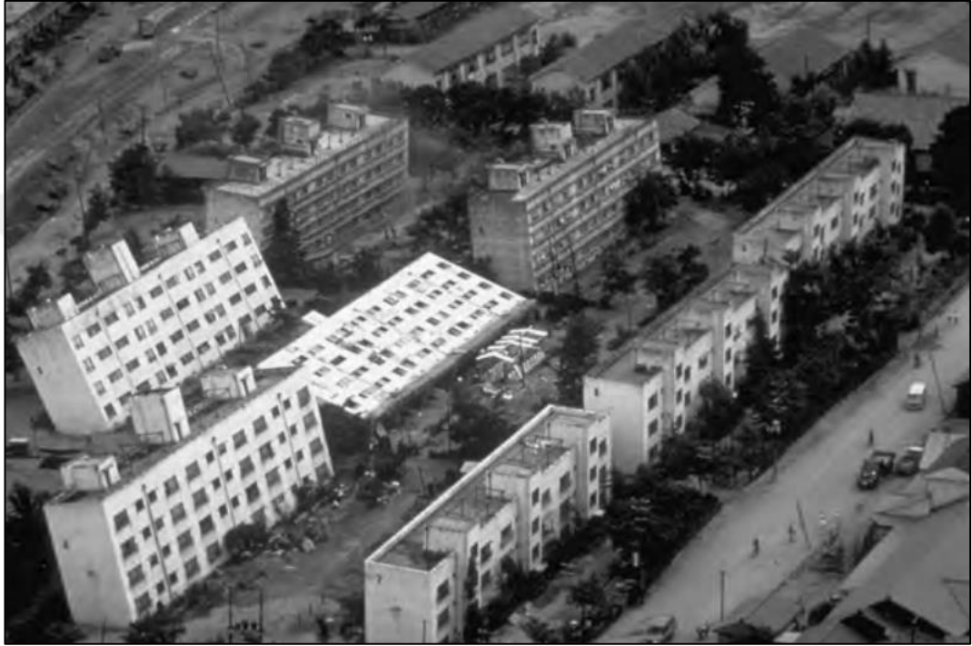
Figure 2.1 Tilting of apartment buildings caused by the 1964 Niigata earthquake (I.M. Idriss & R. W. Boulanger, 2008)
