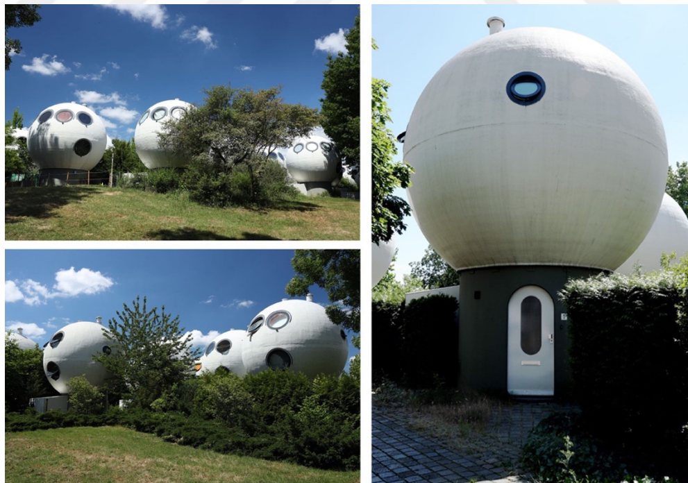
Figure 5 – The Bolwoningen in Maasport, Den Bosch. These spherical houses were designed by Dutch artist and sculptor Dries Kreijkamp and were built in 1984. The 50 houses were originally designed to be made out of polyester, however, fire regulations demanded it to be built from concrete reinforced with fiberglass. Kreijkamp's design is an example to lightweight prefabricated dwelling. (Photographs were taken by the author in June 2020)
