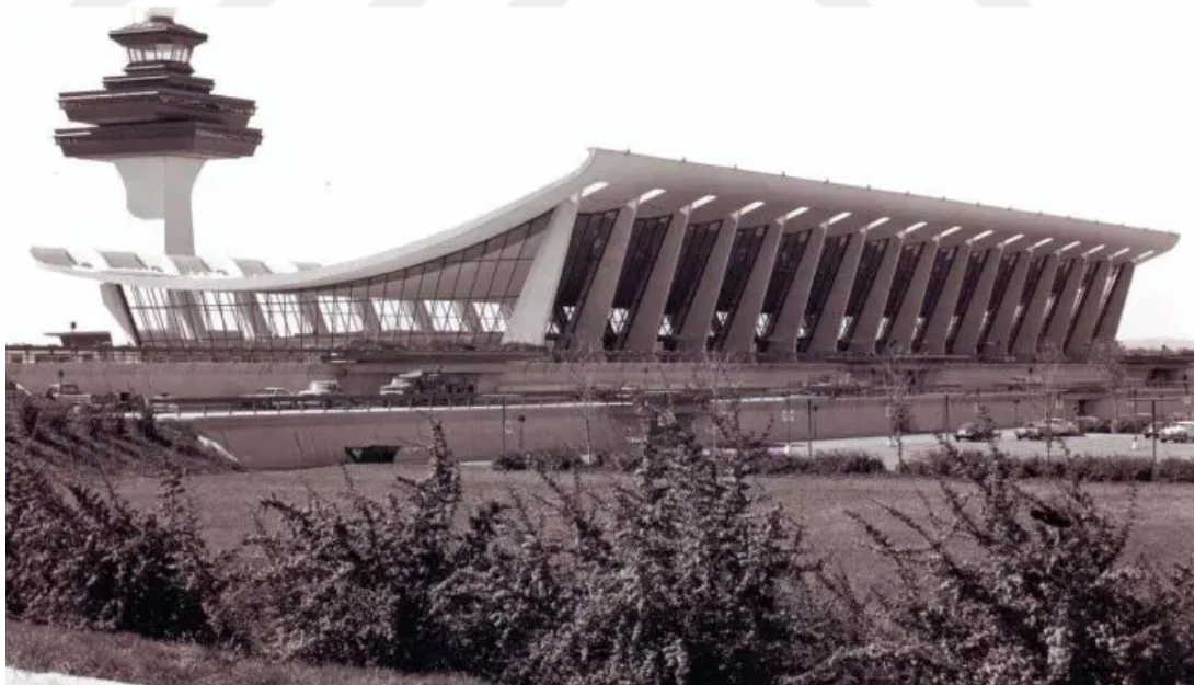
Figure 2 – Dulles International Airport main terminal building in 1962. Note how the terminal could be expanded horizontally from either edge – which eventually did over time. Also note how the overall form of the building is shaped like an aerofoil, alluding the idea of flight. Source: https://seeitsaveit.home.blog/2019/11/19/a-historic-crossroads/
