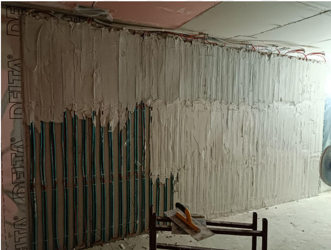
Figure 3.39 PCM wall plastering process
