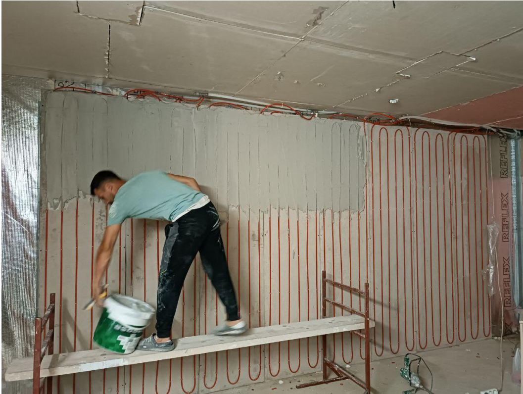
Figure 3.38 Reference wall plastering process
