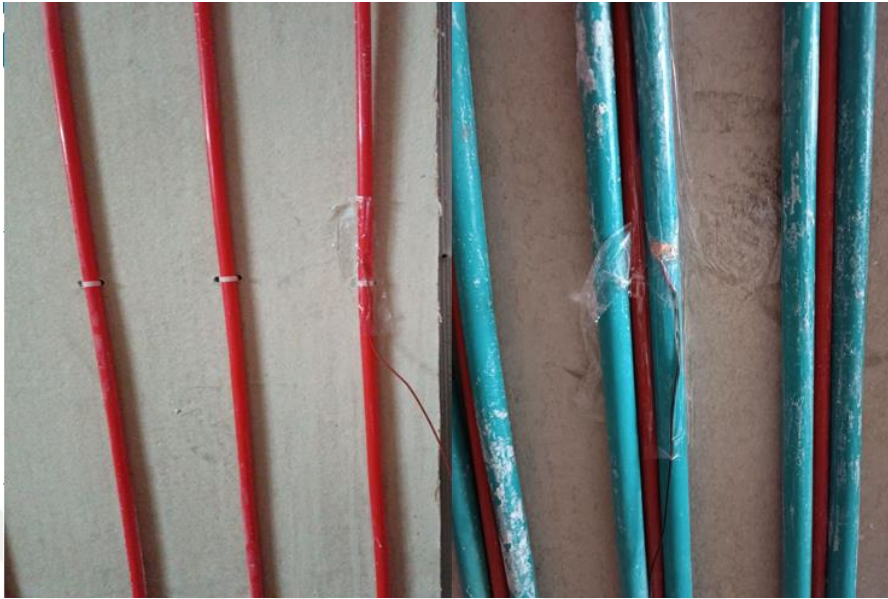
Figure 3.37 Sensor placement image
