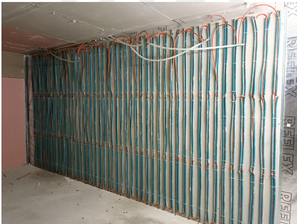
Figure 3.36 PCM wall layout and installation process
