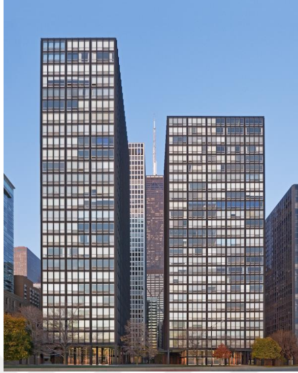
Şekil 3.9: Lake Shore Drive Apartments
