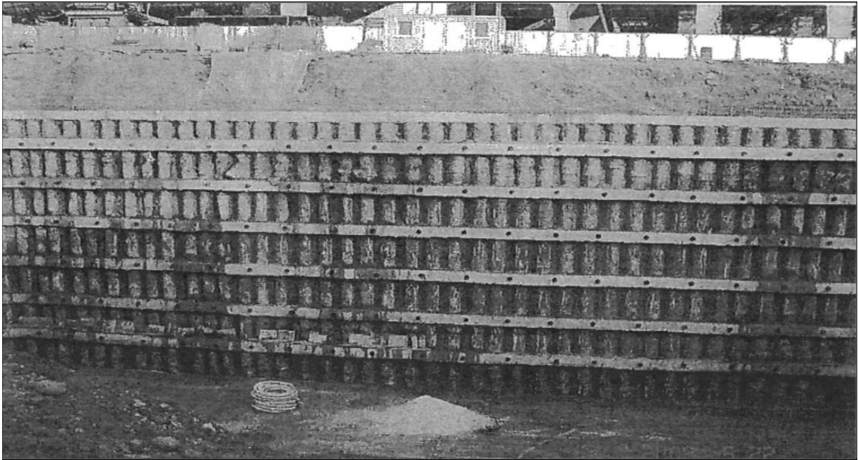
Figure 3.1. A Photograph of the Drilled Shaft Wall (Çalışan, 2009)
