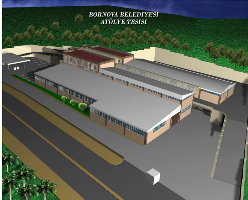
Figure 4.5 Bornova Municipality Warehouse
