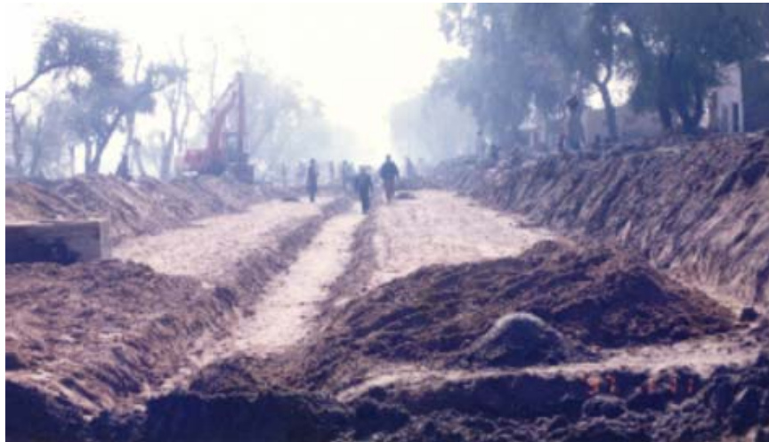
Figure 5.11 Excavation of natural canals to give trapezoid shape.
