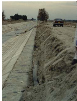
Figure 5.16 Anchoring of geomembrane on the banks before placing of precast units
