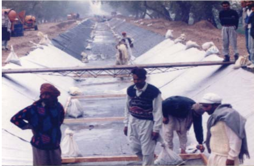
Figure 5.15 Finished form of lined concrete.
