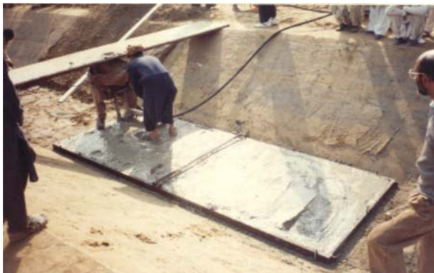
Figure 5.14 Placing of hard cover (in-situ concrete)
