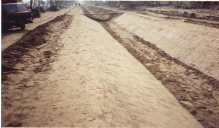
Figure 5.12 Trimming of trapezoidal section to proper shape.
