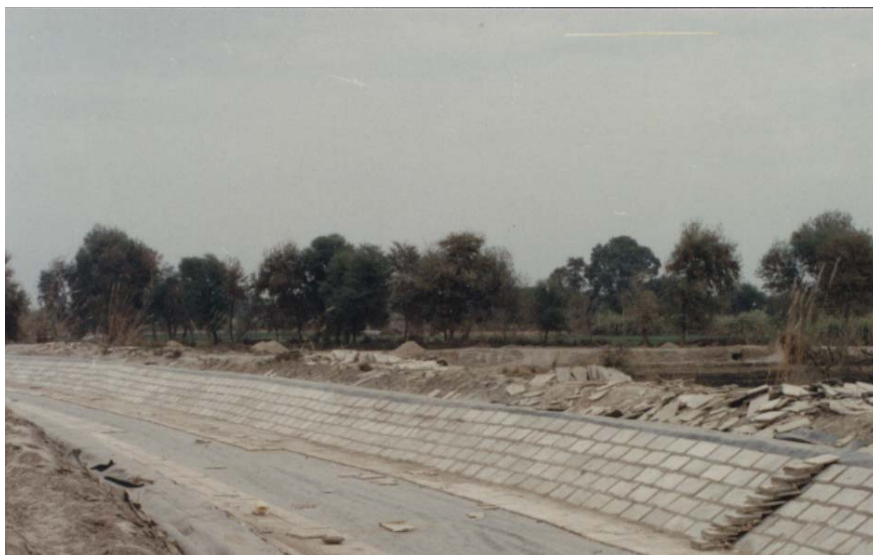
Figure 5.17 Placing of precast units in the canal section
