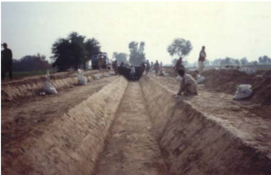
Figure 5.13 Placing of geomembrane before lining.
