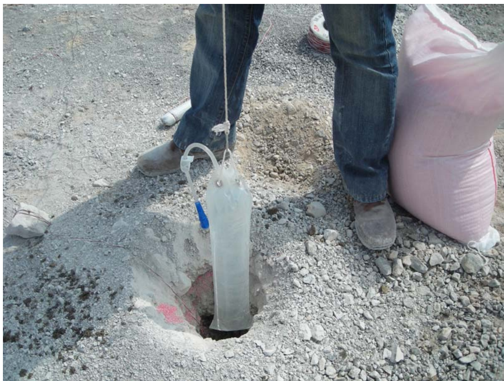
Figure 6.8 Application of water deck by using string with hook
