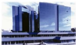
Toprak Center (Business Center)
