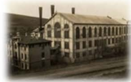
Silahtaraga Electric Power plant
