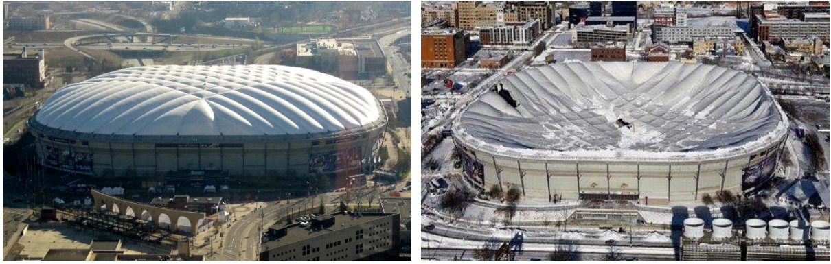
Figure 2.5. Failure of the Metrodome's roof arising from the weight of snow and ice [36].
