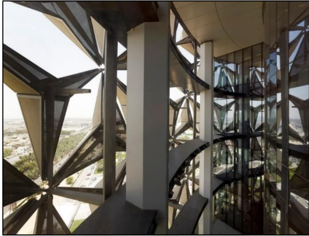
Figure 2.20: A close view of the mashrabiya and curtain wall
