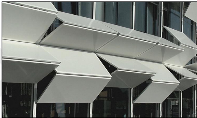
Figure 3.3: Kinetic façade. Kiefer Technic Showroom, Bad Gleichenberg.
