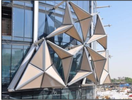
Figure 2.19: Adaptive folding shading system of Al Bahar Towers
