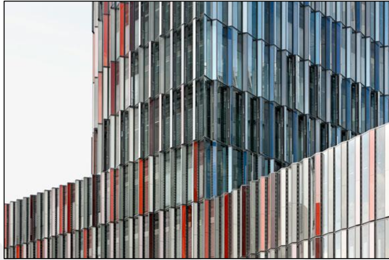
Figure 2.23: Facade detail. KfW Westarkade, Frankfurt.
