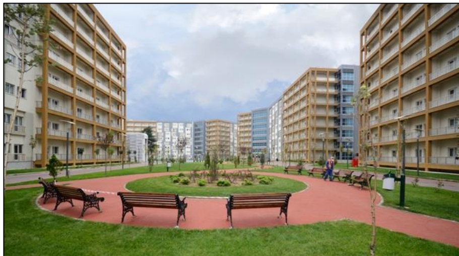
Figure 5.2: Atatürk Dormitory in Zeytinburnu.
