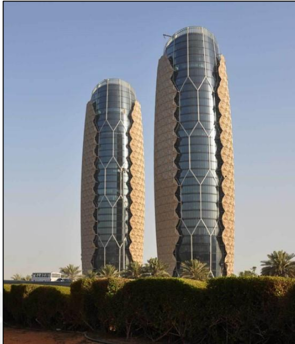
Figure 2.18: Al Bahar Towers
