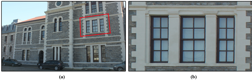
Figure 2.1. Image rectification. a) Original image. b) Rectified area.
