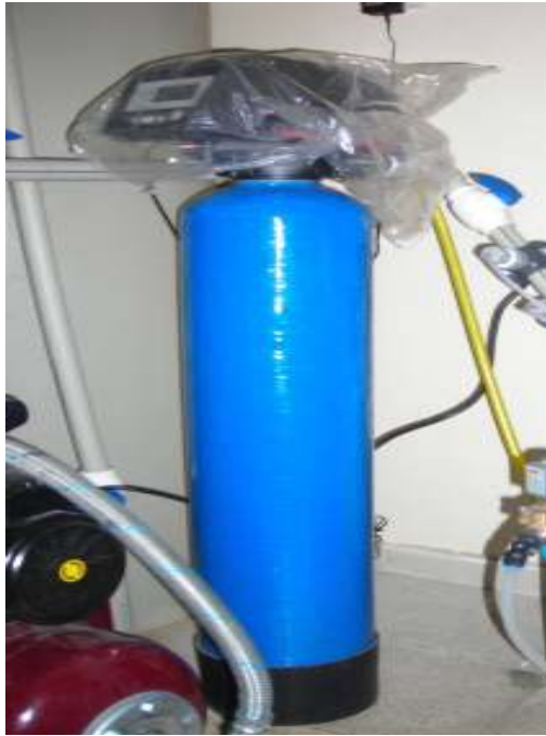
Figure 2.4 Sand filter
