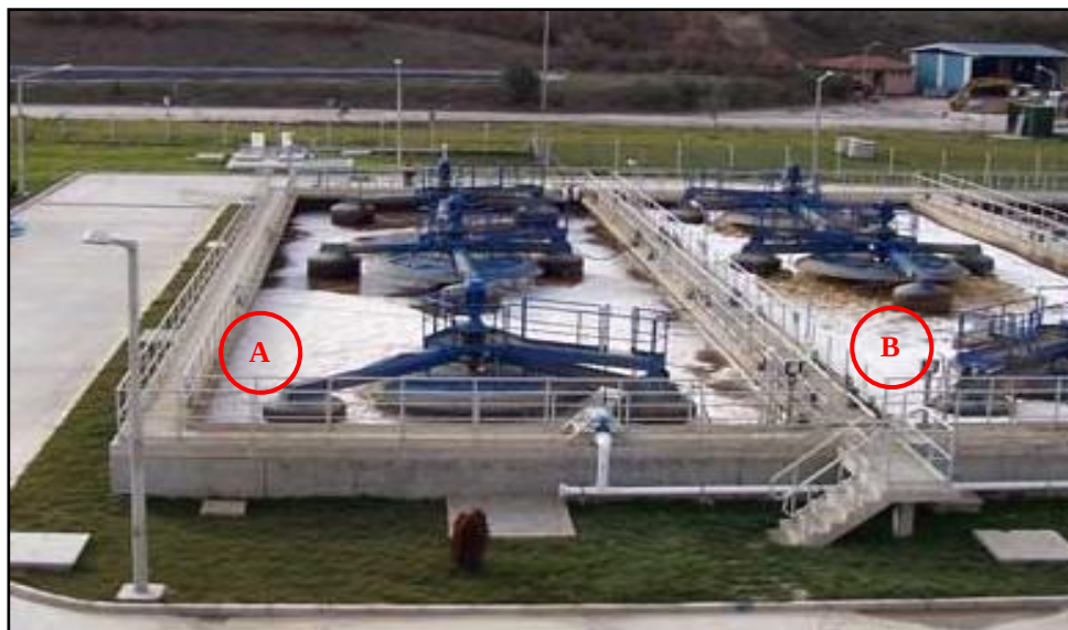
Figure III. 9 Sampling Points of Aerobic Lagoon-1 (A) and Aerobic Lagoon-2 (B)
