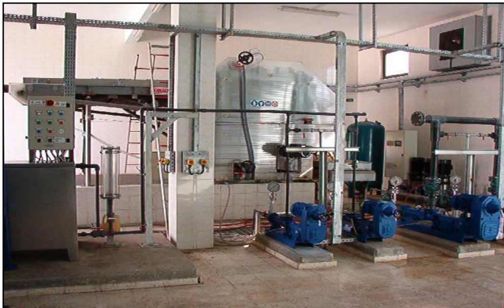
Figure III. 8 Sludge Dewatering System
