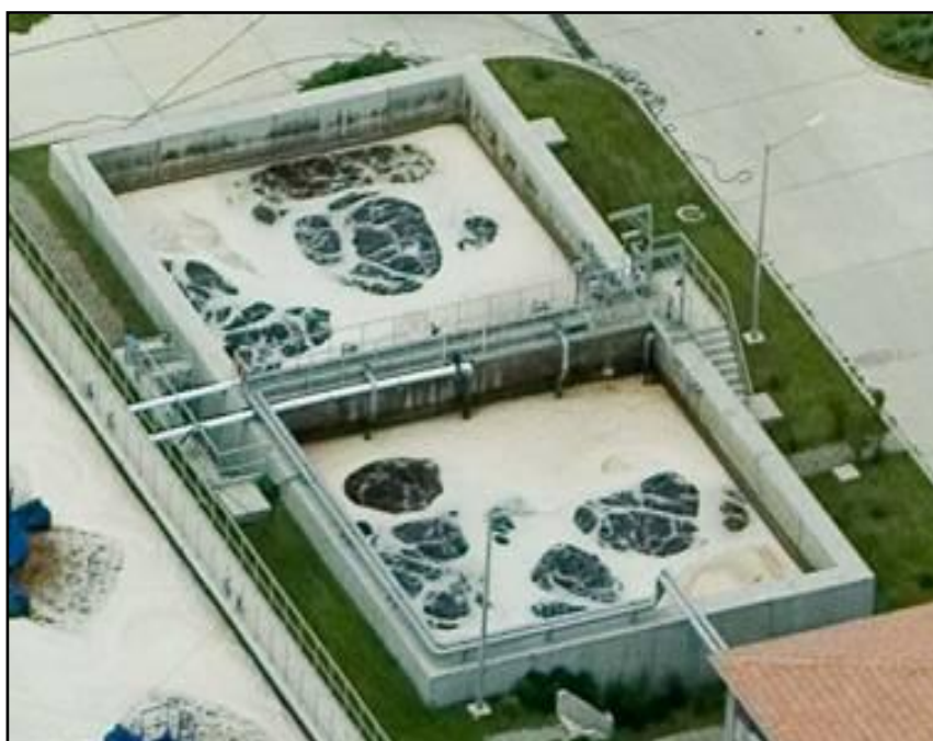
Figure III. 7 Sequencing Batch Reactors
