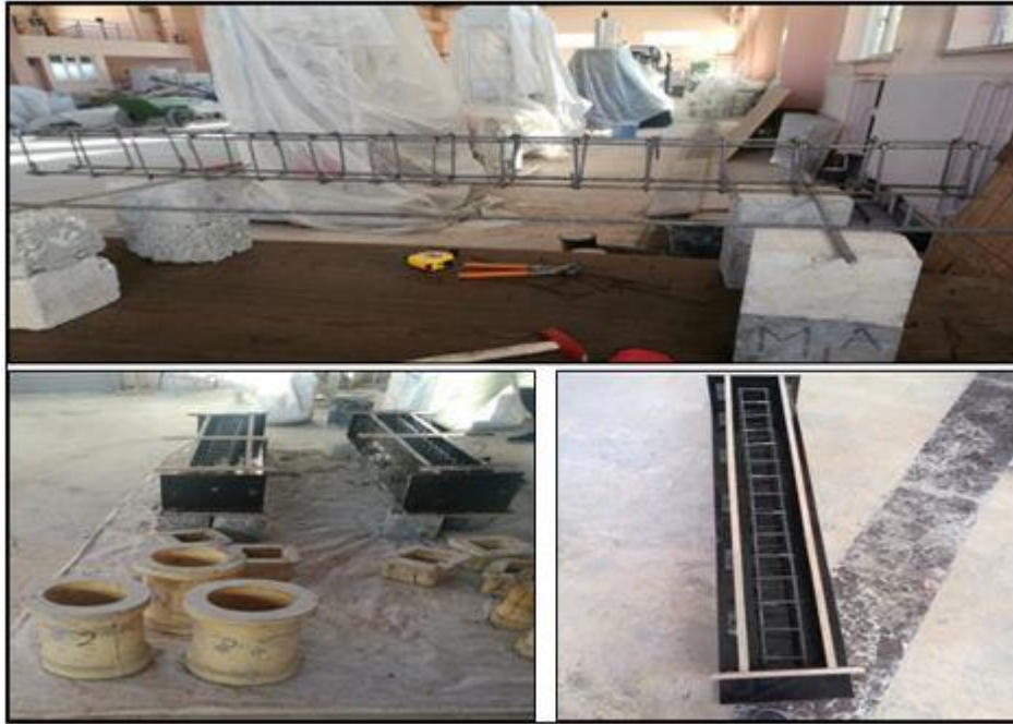
Figure 3.6 Fabrication of reinforcement, greasy and formwork
