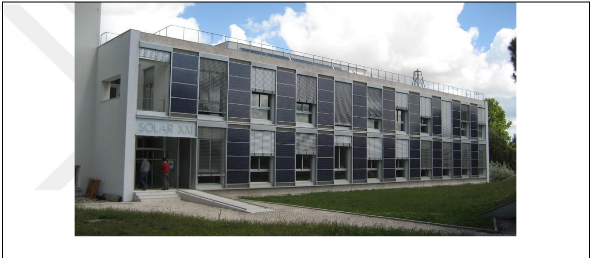
Figure 2.7: The facade of Solar XXI building with PV integrated into its opaque surfaces.
