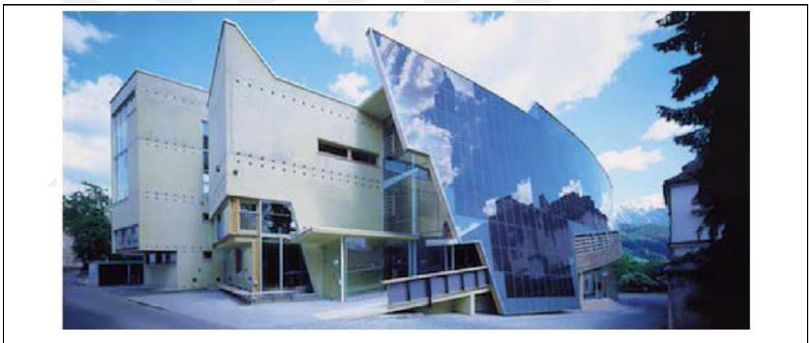
Figure 2.8: Inclined PV integration into the west facade of Vocational College, Austria
