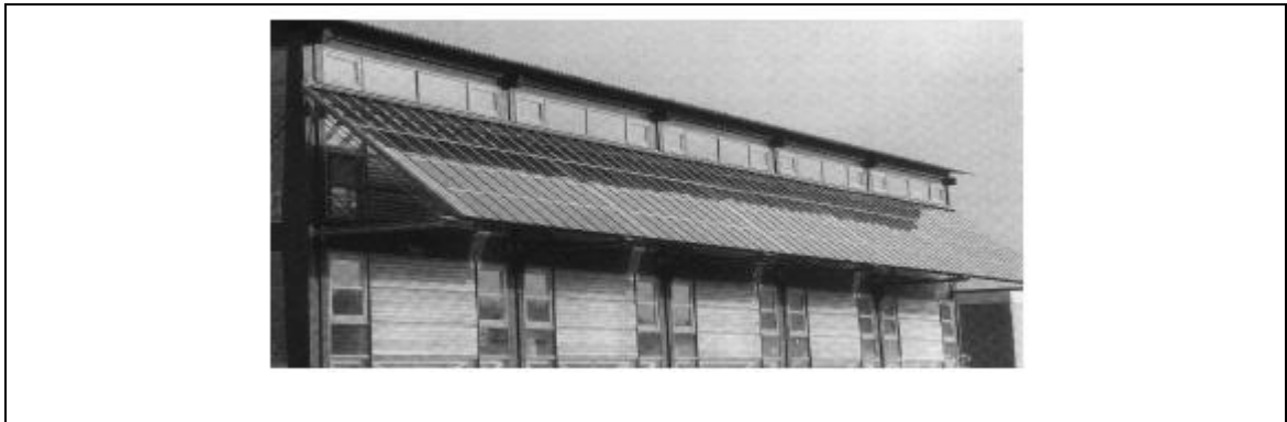
Figure 2.6: An example of solar collectors as shadow devices
