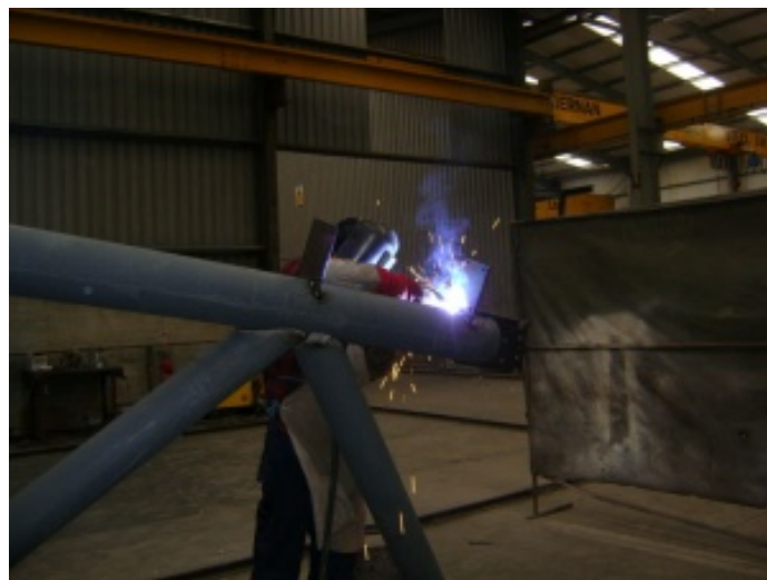
Figure 3.12 : Manual metal arc welding process.
