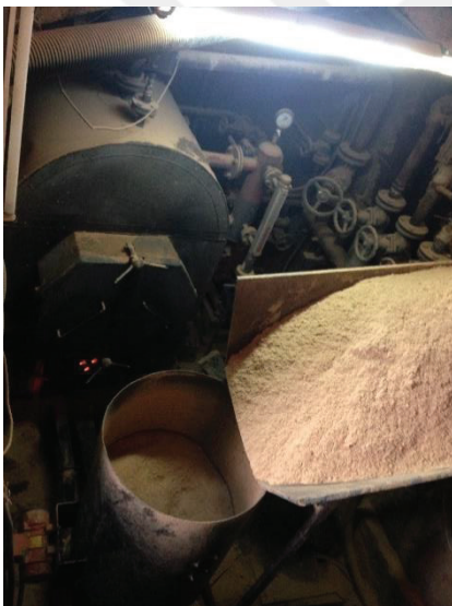
Figure 3.8. Hot Water Boiler.
