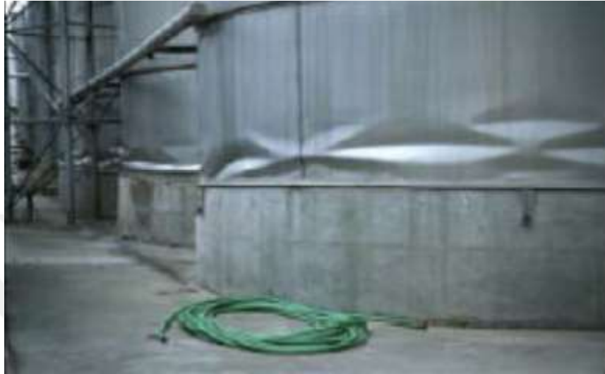
Figure 2.3 Diamond shape buckling.[45]
