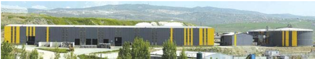
Figure 47 - Anaerobic Digestion Systems (ITC)
