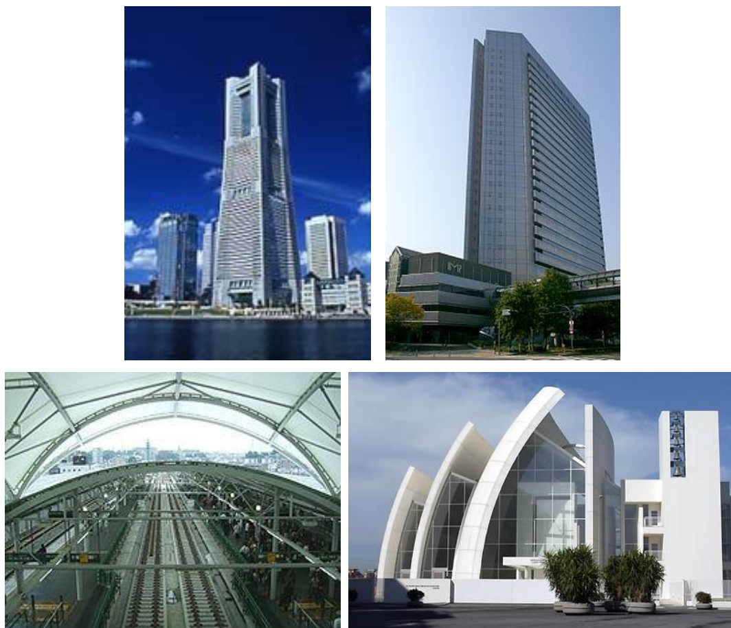
Figure. 1.10. Applications of self-cleaning exterior building materials. Top left to right: MM Towers in Yokohama coated with self-cleaning tiles, Matsushita Denso building covered with self-cleaning glass. Bottom left to right: Self-cleaning roof of a train station in Motosumiyoshi [53] dives in Misericordia Church, Rome, Italy [54,55].
