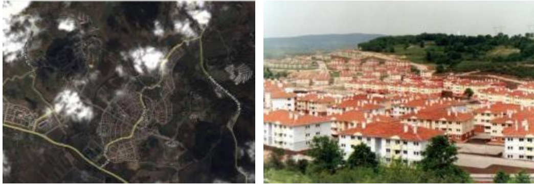
Figure 4.18. Permanent housing district, Adapazarı
