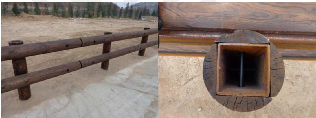
Figure 2.10. Aesthetic timber guardrail reinforced by steel [60].
