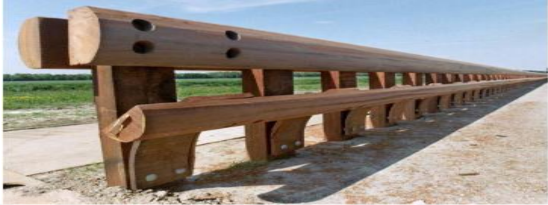
Figure 2.8. Timber guardrail without reinforcing [69].
