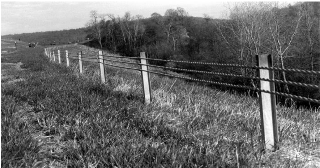
Figure 2.1. Three strand cable barrier [34].
