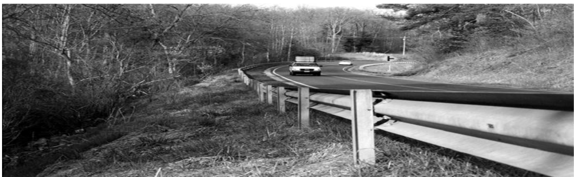
Figure 2.2. W-beam weak post guardrail [34].
