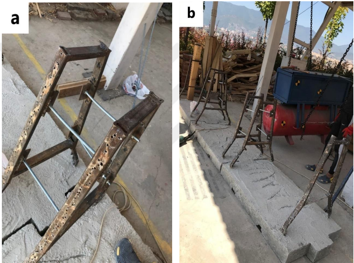
Figure 3.5. (a, b) Connection between metal steels.
