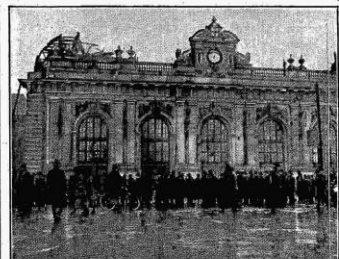
MILAN STATION FIRE. —The ruined central hall of the Central Railway station at Milan after the fire. The big dome of the hall has collapsed. Sparks from a chimney falling on to the wooden roof are supposed to have caused the outbreak.
