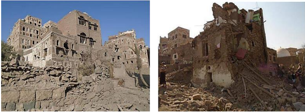
Figure 2.9. Destruction of in the Al-Fulihi neighborhood, Source: Mohanad A. Al-Sayani, 2019.
