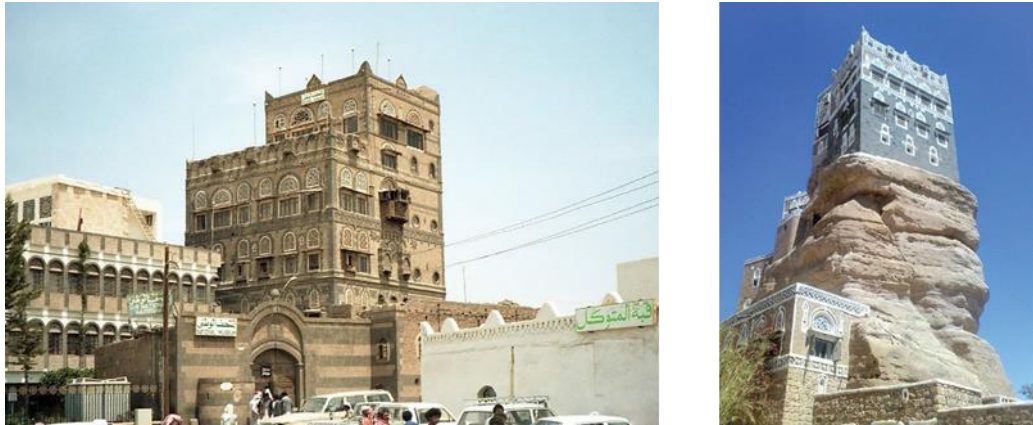
Figure 2.23. The palaces that were built during the Imami rule.
