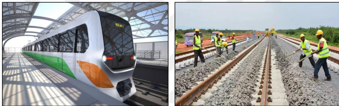
Figure 3.22. Construction of metro abidjan
