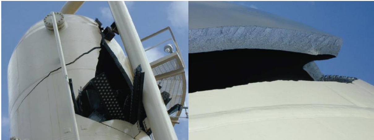
Figure 2.33. Fracture failure of a pressure vessel (Source: https://l24.im/sxS0mTw )
