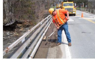
Removing dirt and other debris from the bridge wearing surface.
