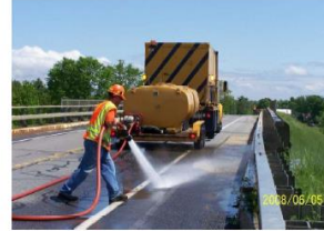
Volume washing the bridge deck.
