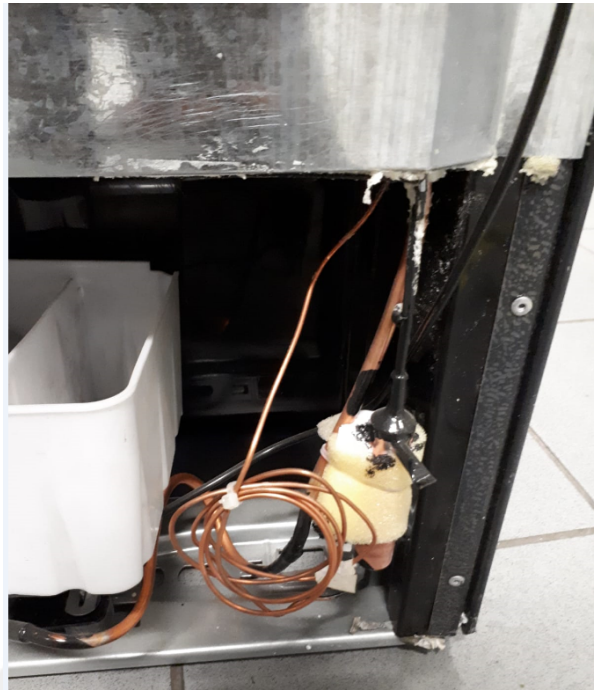
Figure 6.5. Capillary tube.
