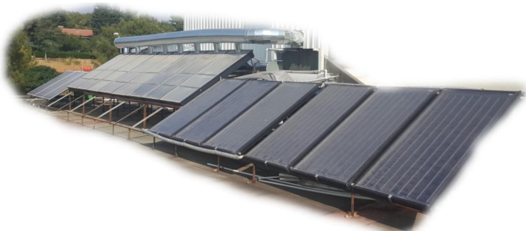
Figure 3.4 Solar panels of solar drying system
