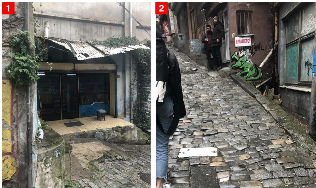
Figure 4.13. Public bath (left) and left luggage office (right) located in Alageyik Street (Source: Personal archive, 2020)
