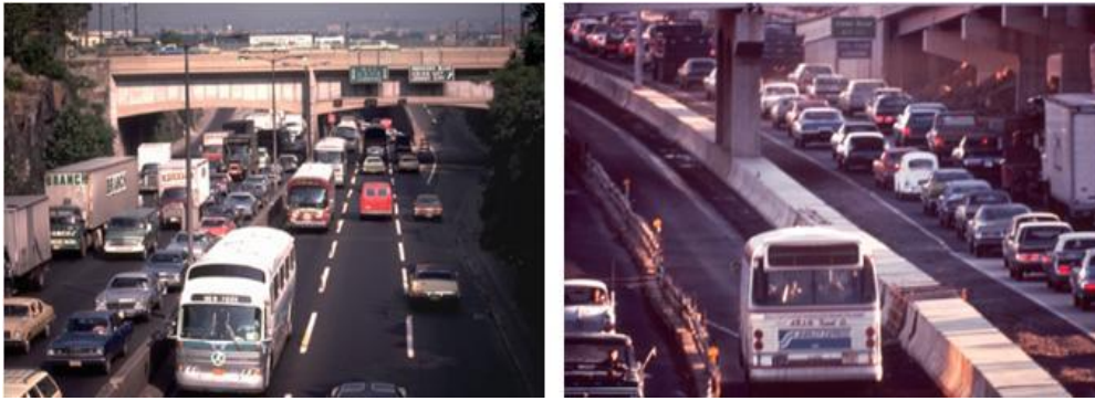
Figure 2.2 : Early bus-only lanes on freeways in the US.
