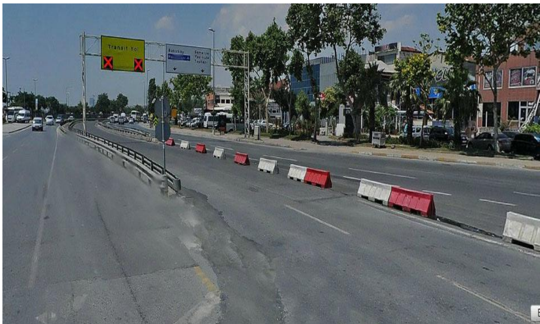
Figure 3.7 : Beginning of reversible operation in Yenikapı.
