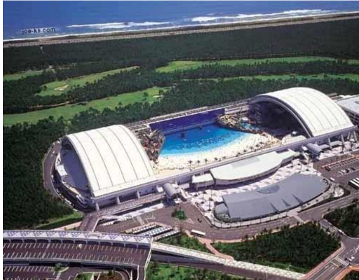
Figure 3.46. Ocean Dome Miyazaki City, Japan (Gantes, 2001)
