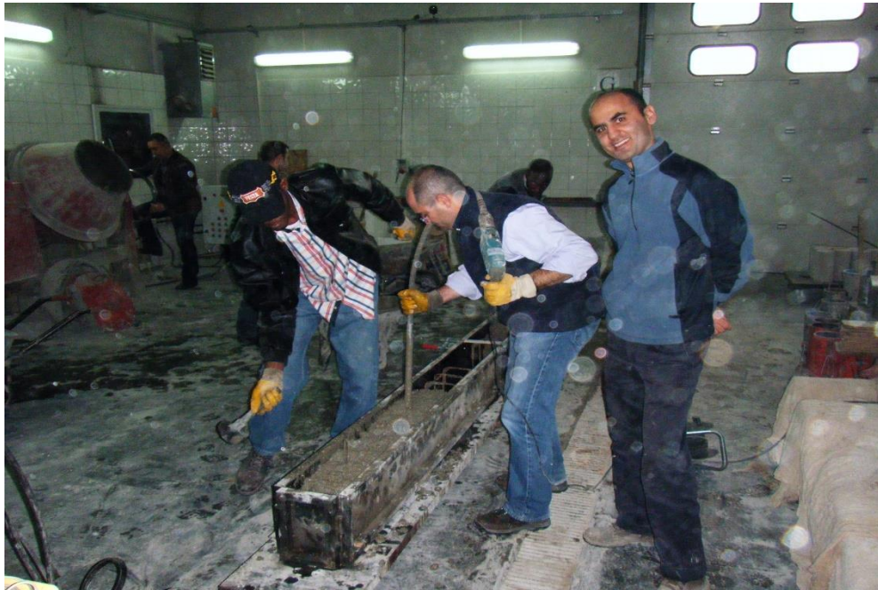
Figure 3-7 – Placing concrete in formwork
