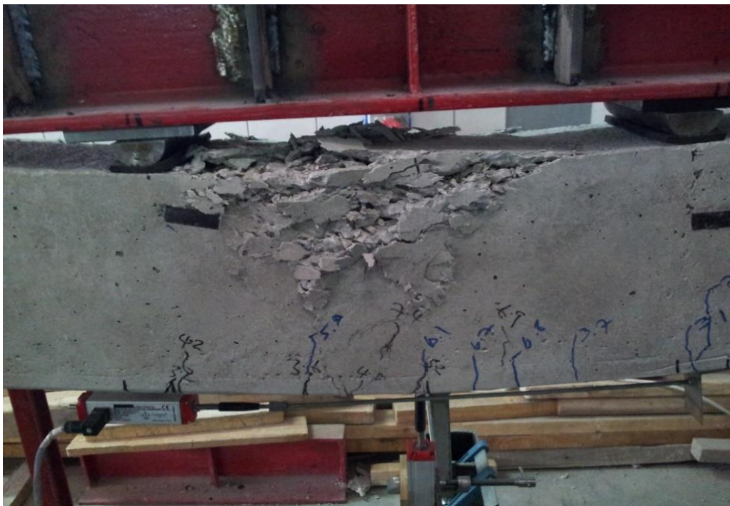
Figure 4-6 – Failure and crack pattern in SFRC Beam 3φ18 ( \rho = 2.02\% )
