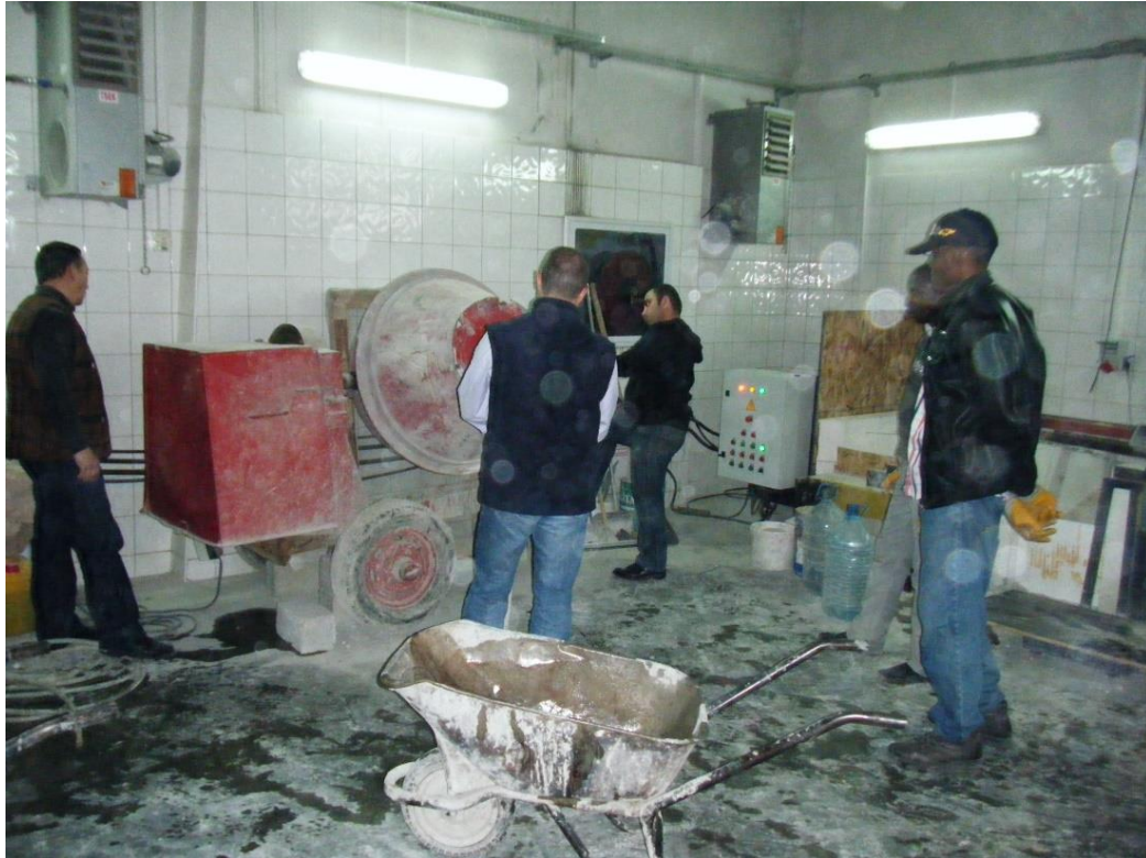
Figure 3-6 – Mixing of materials in progress
