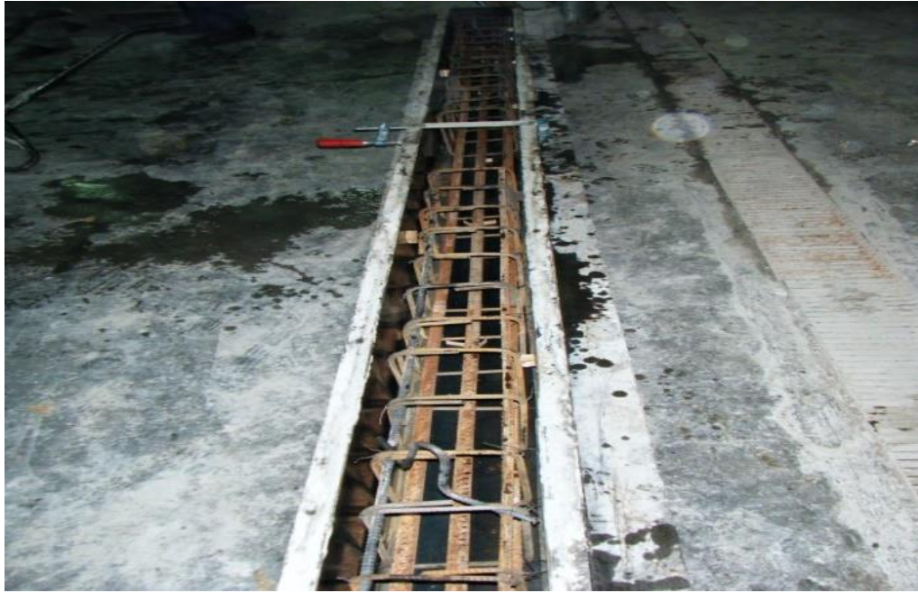
Figure 3-5 – Reinforcement cage in the formwork
