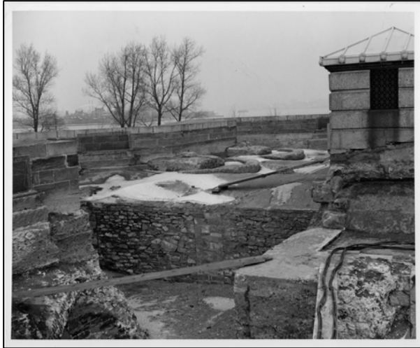
Fig.2.4. Photo of the excavation undertaken for the construction of the American Museum of Immigration, 1961 Photograph Collection of the American Museum of Immigration, Liberty Island, U.S., Department of the Interior, NPS.
