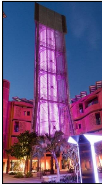
Figure 5.12: Wind Tower lighting (D'Eramo, A, 2021, 10)
