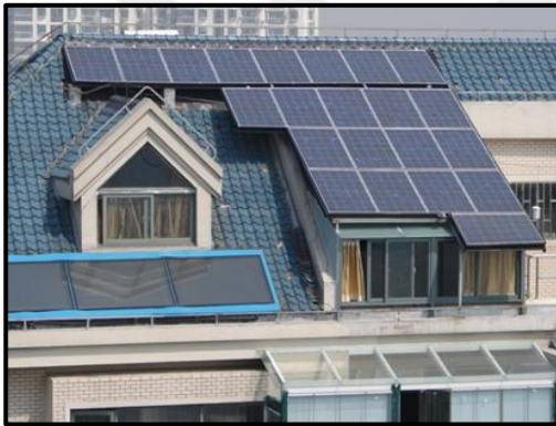
Figure 4.11: BIPV Pre-installation design (SRNE, 2021).
