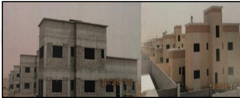
Figure 6.16: The construction phase of Al Falah Complex Housing (Bande, L, et al., 2019, 4).
