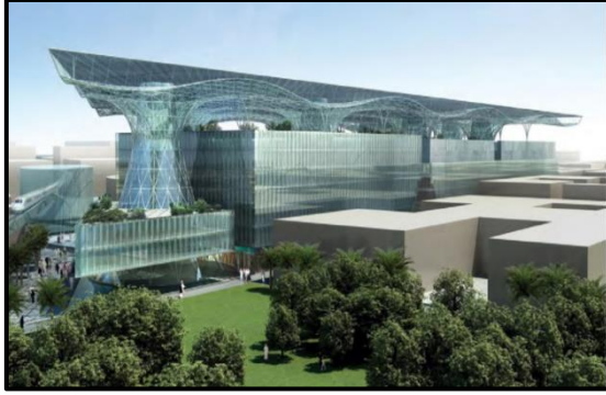
Figure 6.10: Main structure in Masdar city (Elgendy, K, 2010)
