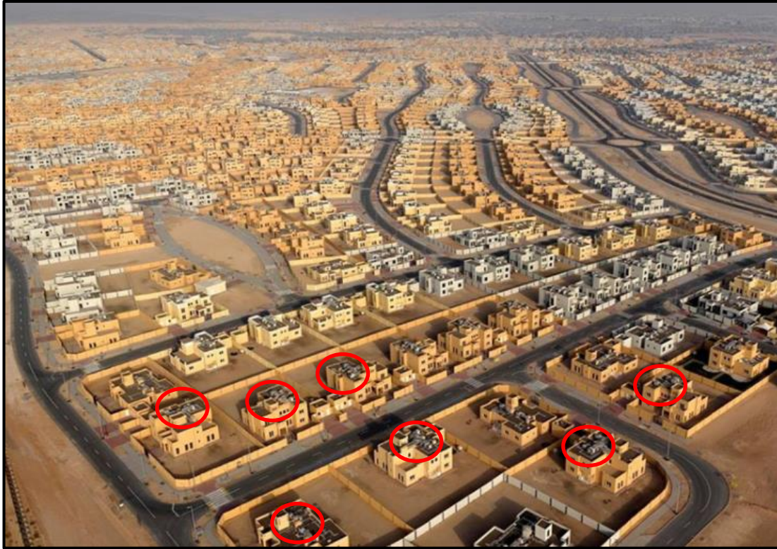
Figure 6.19 : Solar collectors on the roofs in the Al-Falah city (Al Akayleh, A, 2011)
