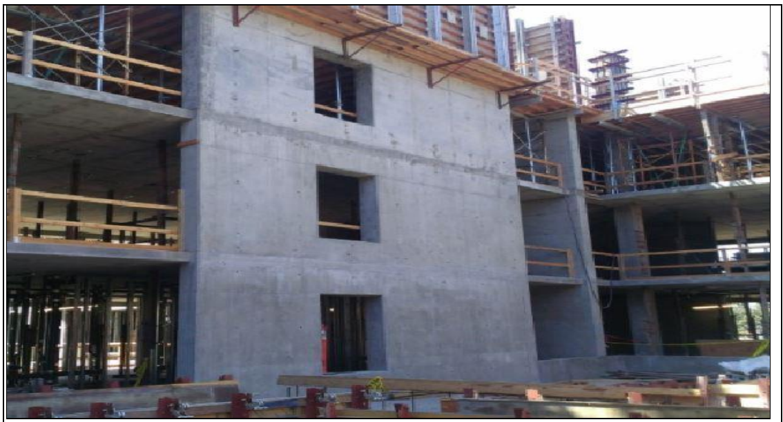
Figure 2.1b: Shear Wall Cast in the Construction Site ( https://structville.com/2020/10/bracing-systems-in-a-high-rise-building.html )
