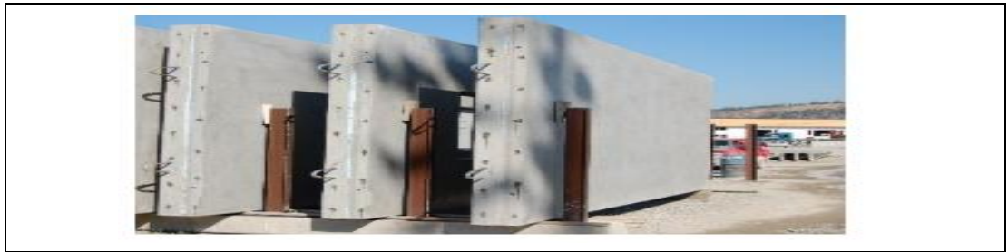
Figure 2.2: Concrete Shear Wall ( https://www.thestructuralworld.com/2018/09/08/concrete-shear-wall-design/ )
