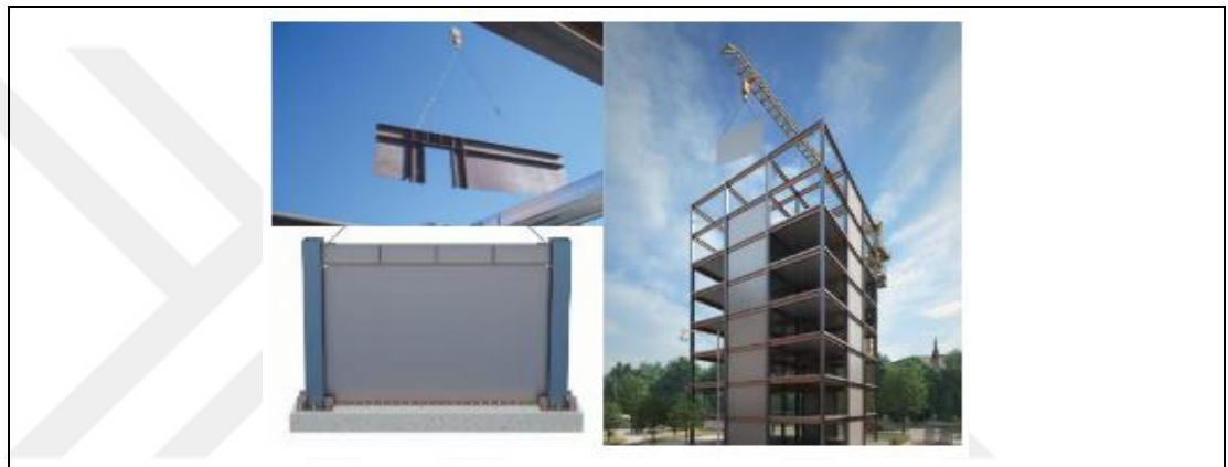
Figure 2.3: Steel Shear Wall ( https://www.canadianconsultingengineer.com/features/steel-plate-shear-walls/ )
