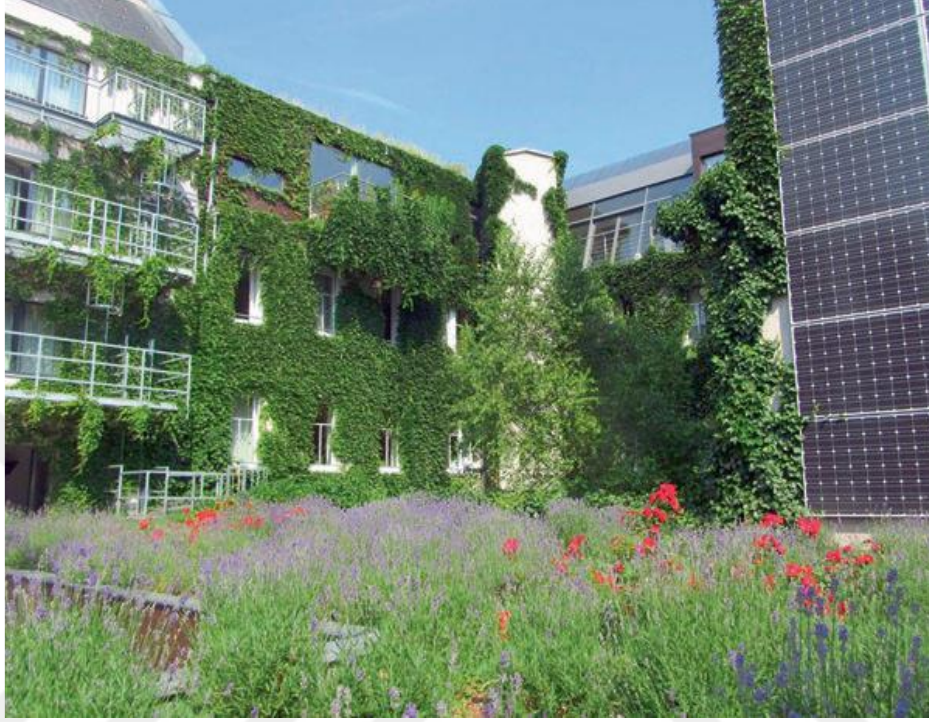
Şekil 2.24 : Zero-emission Boutique Hotel Stadthalle, Vienna (Enzi vd., 2017).
