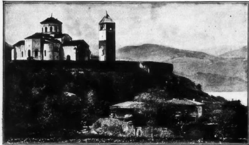
Şekil 4.45. Trabzon Ayasofya Camii, 1899 (Dulany Hunter, The Princess of Trebizond)
