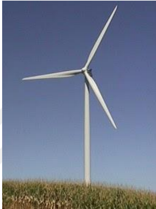
Figure 2.2 Horizontal Axis Wind Turbine (Sebit, Alpman and Yılmaz 2014).
