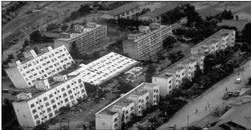
Figure 1.3: Sloping of the buildings by the 1964 Niigata earthquake [1].
