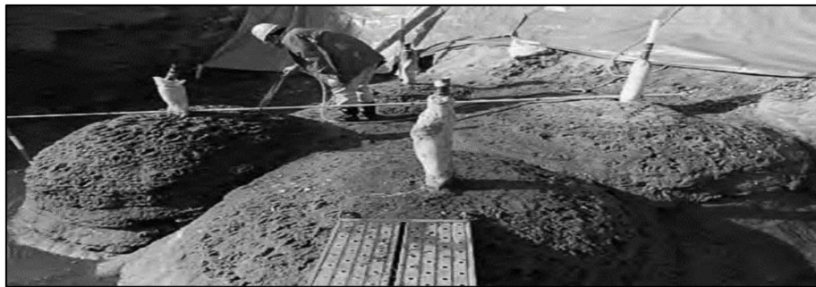
Figure 1.10: The permeation grouting method [1].
