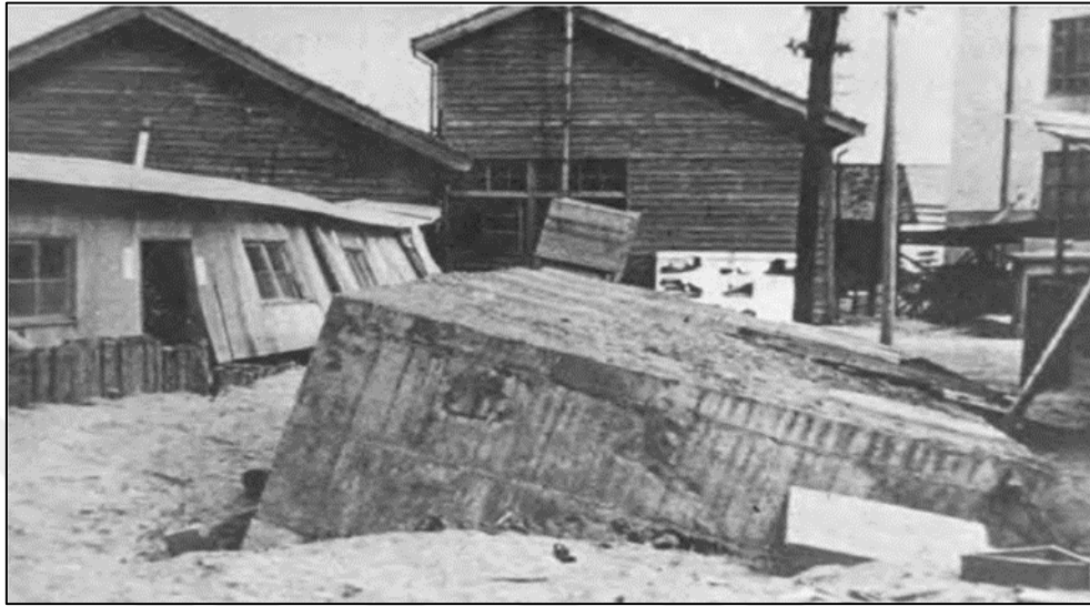
Figure 1.2: The uplifting of buried tank in liquefied soil by the 1964 Niigata earthquake [1].
