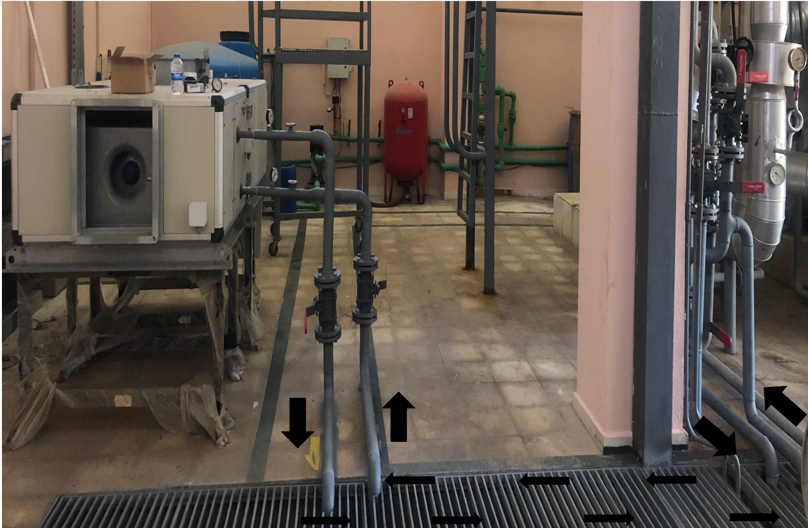
Figure 4.8. Dryer-geothermal line connection
